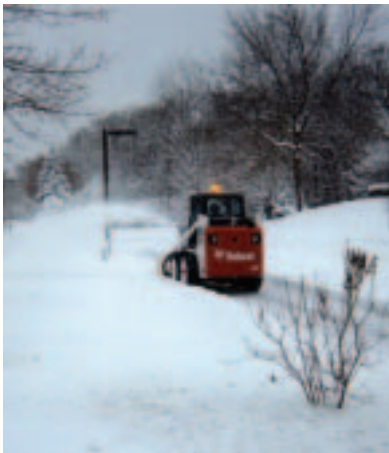
The crew gets out early to clear roads and walkways.
